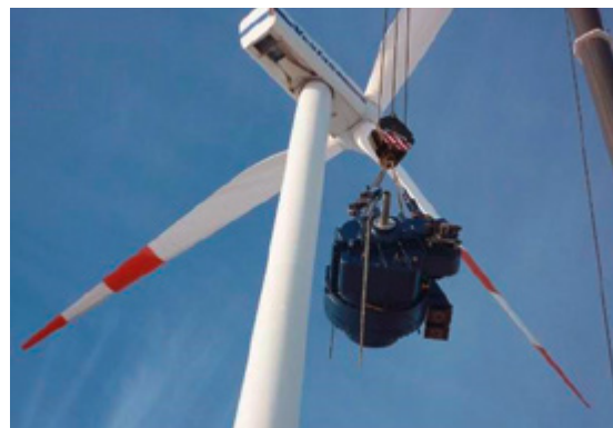
Figure 35: Replacement of the gearbox, without dismantling of the rotor; source: R+V
