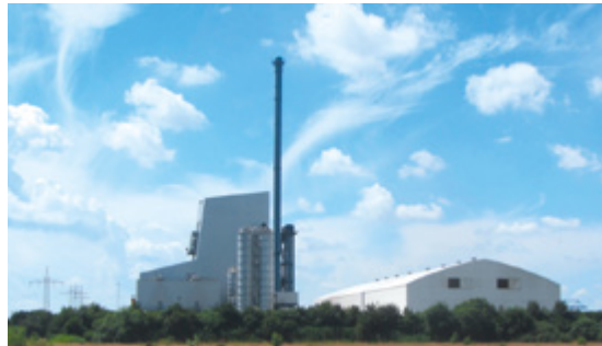
Figure 1: Biomass power station with adjoining raw material storage; source: VGH
