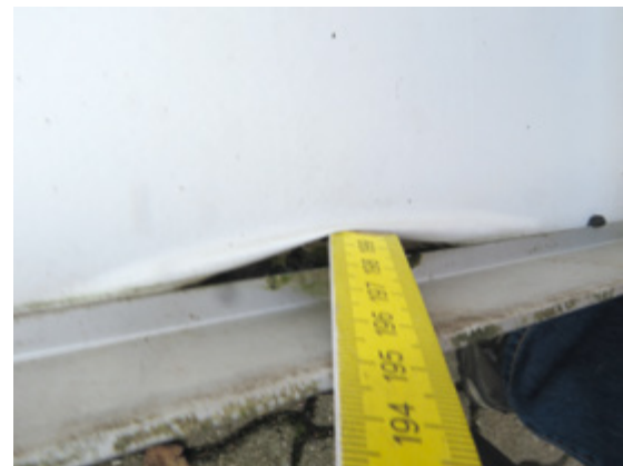
Figure 6: Delamination; source: PVGutachten.info
