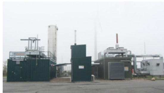
Figure 3: Amine scrubbing for methane treatment (left); source: VGH
