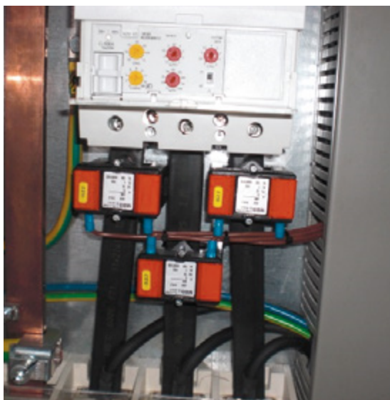
Figure 38: Load-break switch; source: VGH
