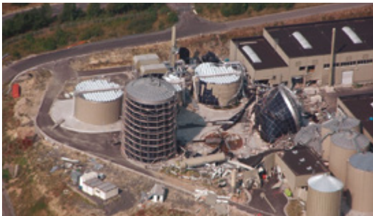
Figure 33: Leaked biomass/substrate; source: VGH
