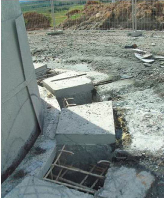
Figure 46: Restoration of a foundation; source: Gothaer, Edgar Sensen
