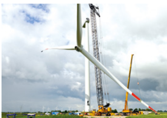
Figure 10: Mounting of a rotor; source: Senvion GmbH
