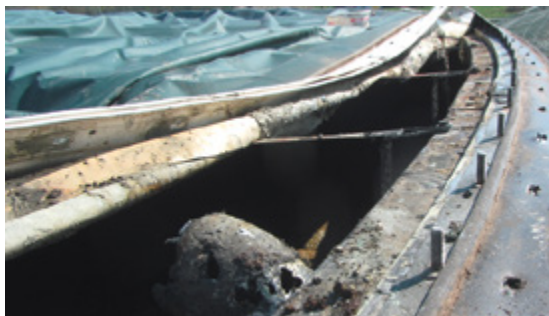
Figure 16: Concrete tanks; source: VGH
