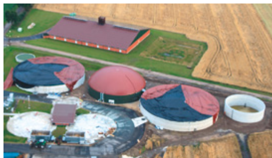
Figure 15: Storm damage ~100,000 euros; source: R. Evers
