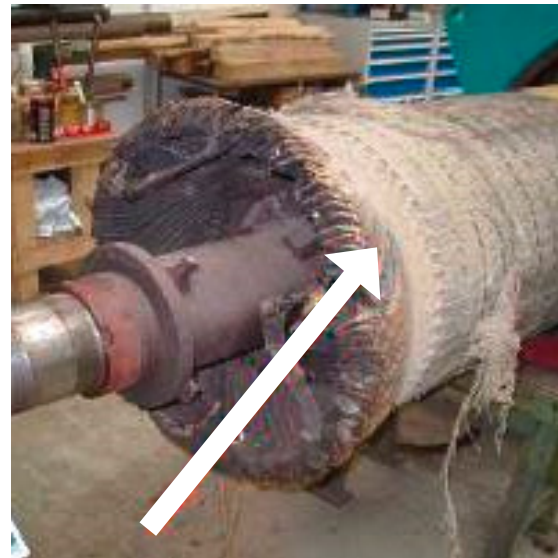
Figure 36: Fanned out winding of a slip ring rotor due to a torn rotor bandage; source: Allianz
