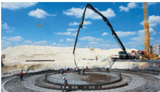
Figure 5: Construction of a foundation; source: Enercon GmbH
