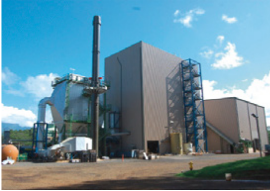
Figure 5: Biomass power plant; source: Teko
