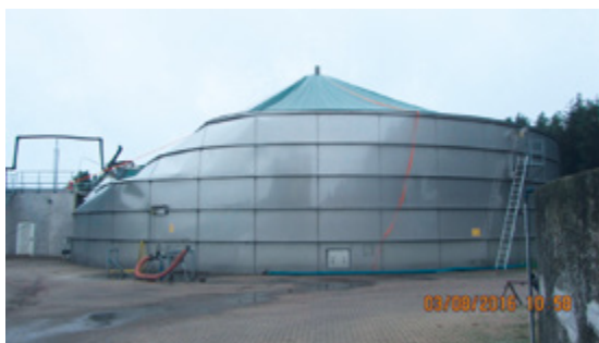
Figures 18–19: Dented container, damage costs: 200,000 euros; source: VGH
