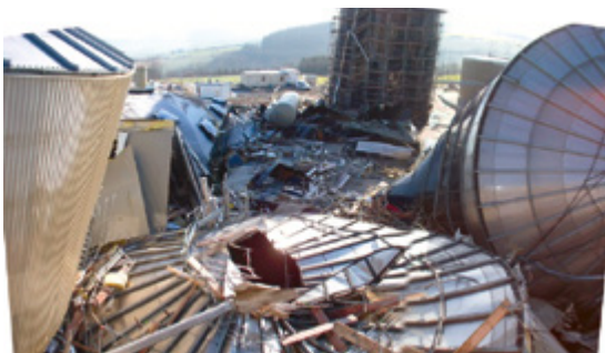
Figures 34–35: Tank rupture after refilling; source: www.as-nds.de
