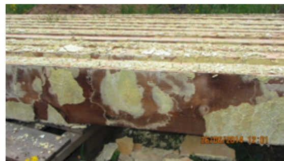
Figure 13: Sulfide deposits; source: VGH
