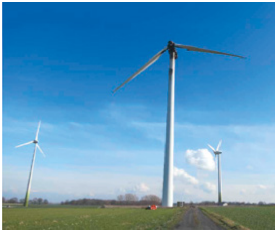
Figure 2: Wind turbine damaged by fire; source: Teko
