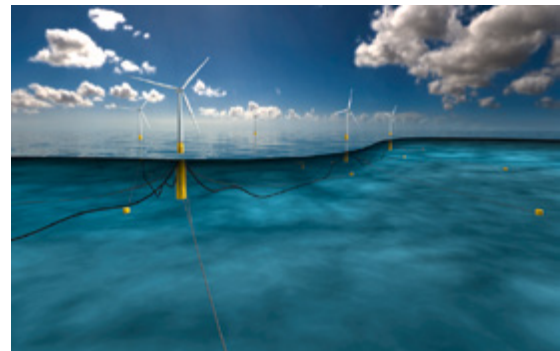
Figures 56–57: A floating wind energy plant at Project Hywind off the Norwegian coast; source: Statoil
