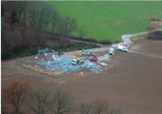
Figure 1: New high voltage mast; source: Teko
