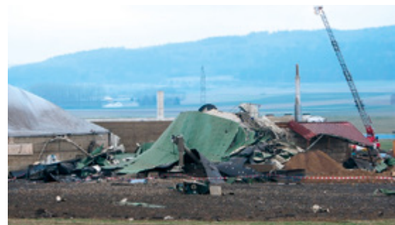
Figures 36–37: Tank rupture after commissioning; source: Thomas Warnack
